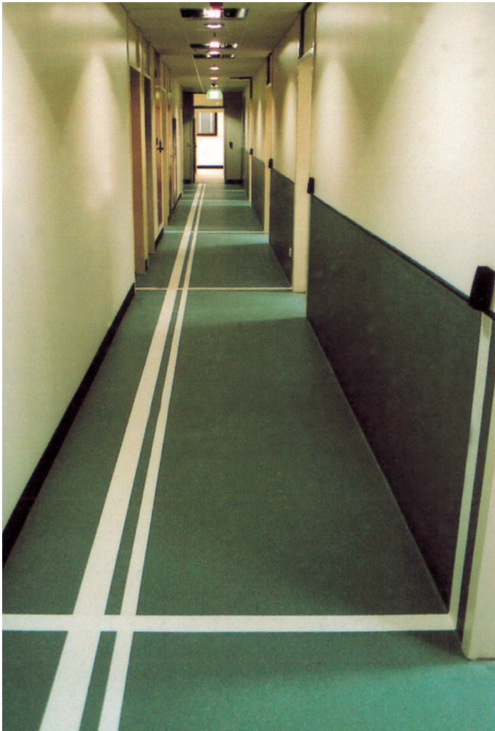
Cap Seal installed in conjunction with "Futura" rubber flooring from Spectrum Floors
